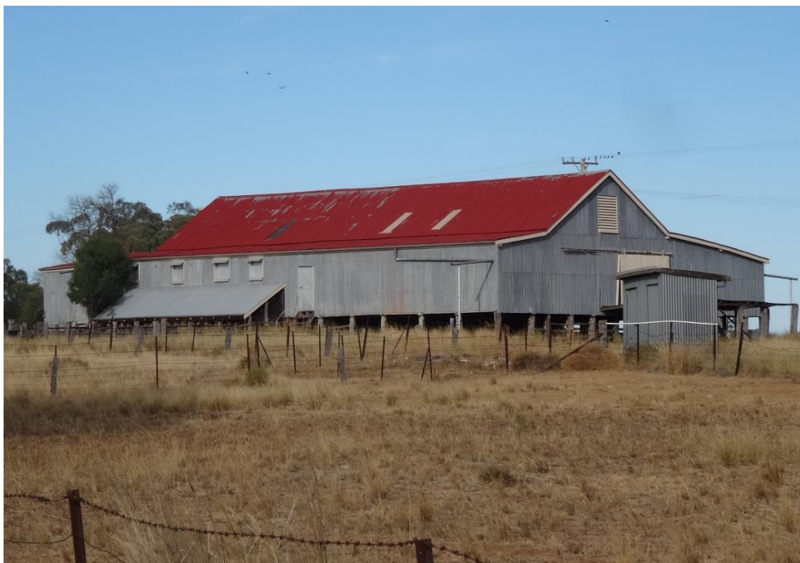
Figure 21. View facing the rear elevation of the shearing sheds forming part of the Kurrumbede Complex (Site 9).
