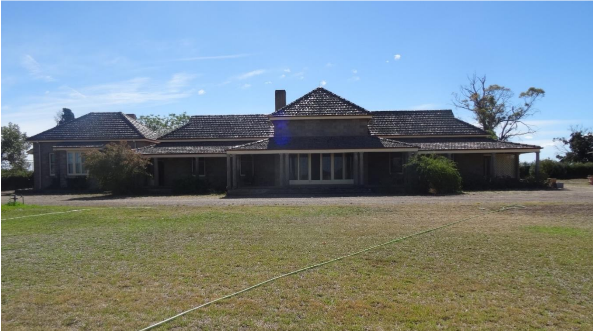
Figure 12. View facing north towards the front (south) elevation of Kurrumbede Homestead. The nearest piece of visible Project infrastructure, not including the Project rail spur, would be the Project CHPP, approximately 830 m to the north-east beyond the homestead in this image.
