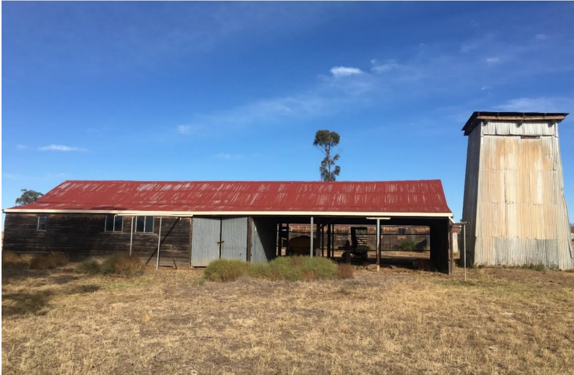
Figure 16. View facing south of a hay silo and work shed north of the homestead and forming part of the Kurrumbede Complex (Site 4). The nearest piece of Project infrastructure, not including the rail spur, would be a dam approximately 550 m beyond the structures in this image.
