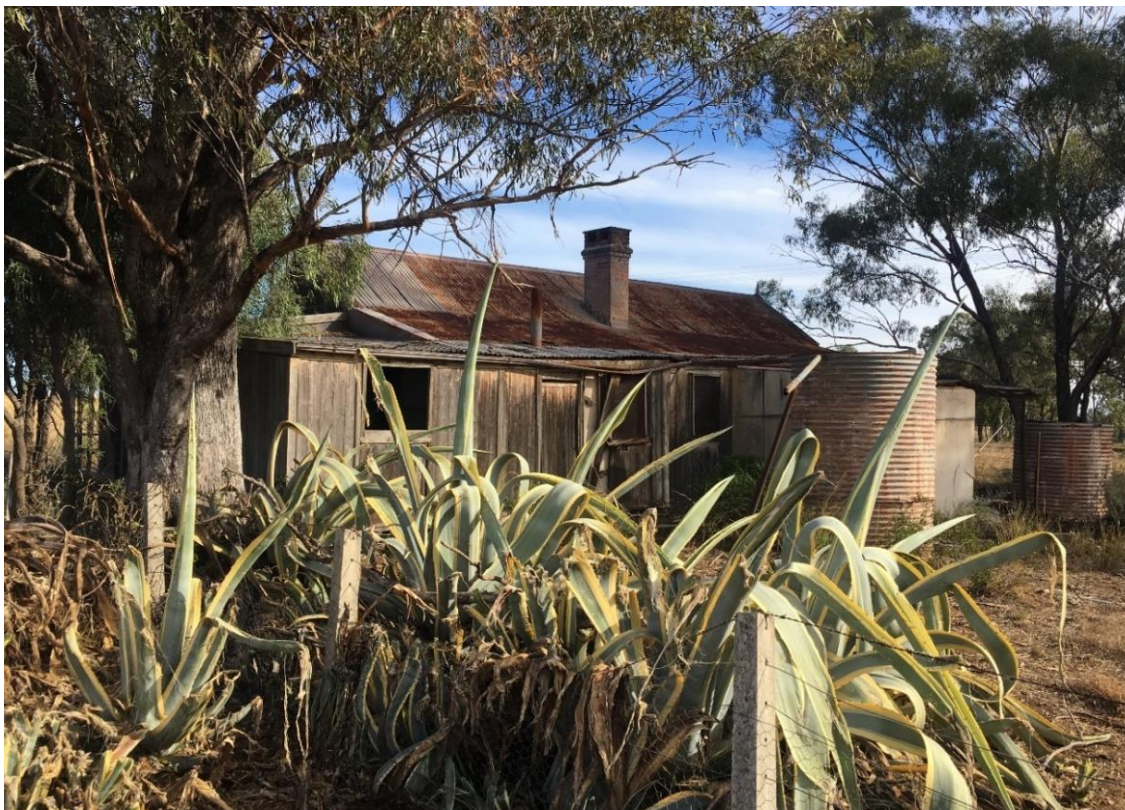
Figure 15. View facing south-west of one of the weatherboard cottages north of the homestead and forming part of the Kurrumbede Complex (Site 3).
