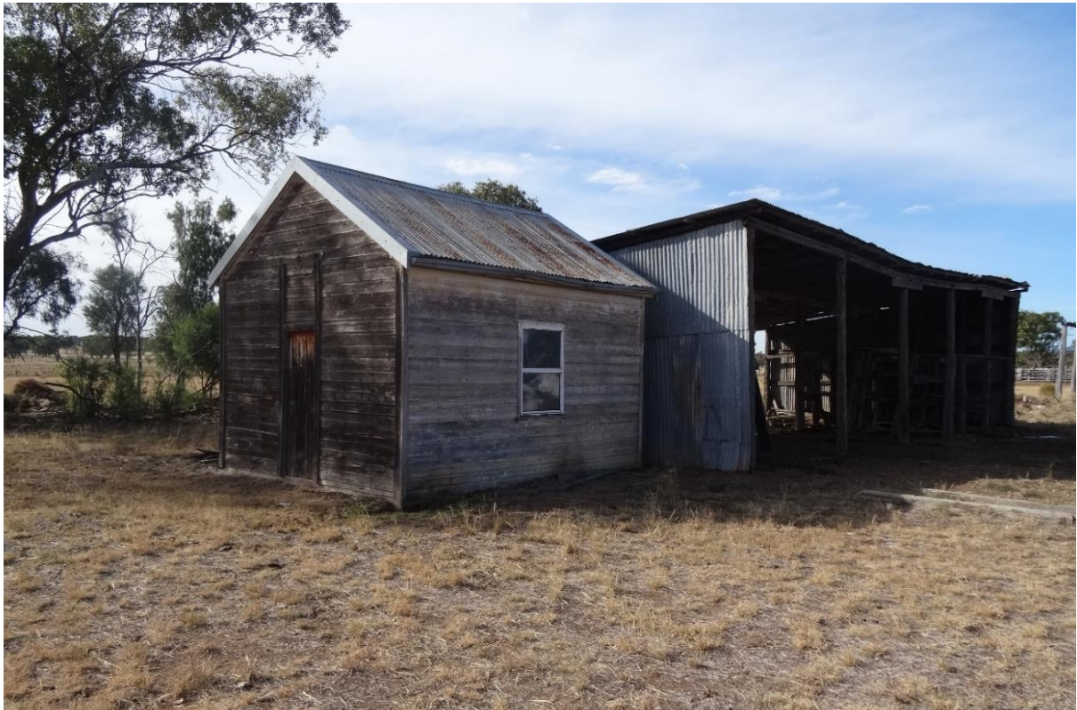
Figure 18. View facing north-east of a timber work shed forming part of the Kurrumbede Complex (Site 6).
